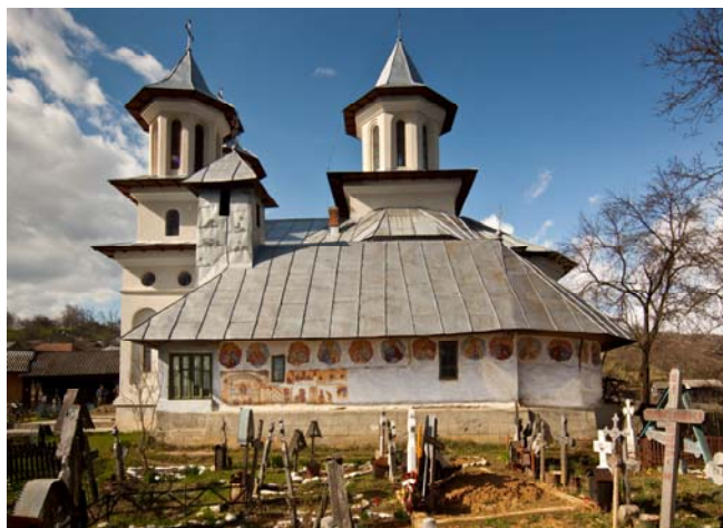
Fig. 1a – Holy Trinity Church from Urechești-Cicanești (in the background a modern brick Church).
